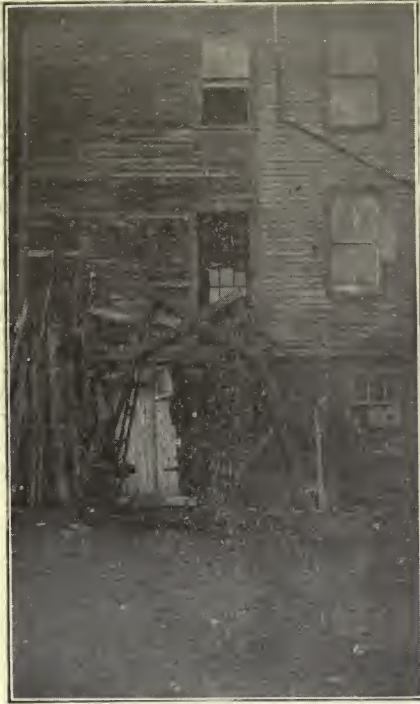
Through the doorway may be seen the window of a semi-dark room, deriving its only light and air from the hall
